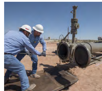
↑ Lucid pipeline operating team members remove a pipeline pig from infrastructure following a cleaning operation ← Red Hills teams maintain the integrity of the assets located at the largest gas processing complex in the Delaware Basin
